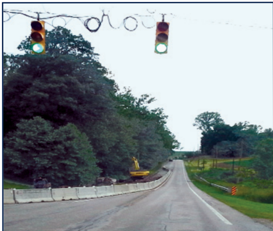
Signalized one-lane, two-way long-term control (Source: N. Carboneau).
