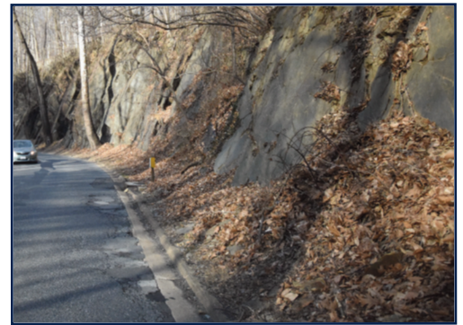
A section of road that restricts flagger and sign placement (Source: FOF).
