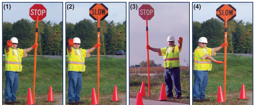
Positioning the single flagger off of the shoulder with cones, as shown, for added delineation is a good practice (Source: N.Carboneau).
