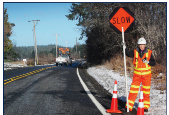
Flagger station with a pilot vehicle leading traffic (Source: Washington State DOT).
