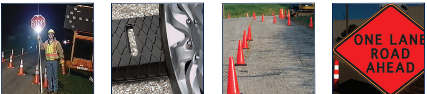
Examples of countermeasures to alert drivers (left to right): Stop-slow paddles with supplemental lighting and an arrow board, rumble strips, additional centerline channelizing devices, and larger fluorescent signing with high retroreflectivity values (Sources: Michigan DOT, Plastic Safety Systems, N.Carboneau, and Spark 3M News).
