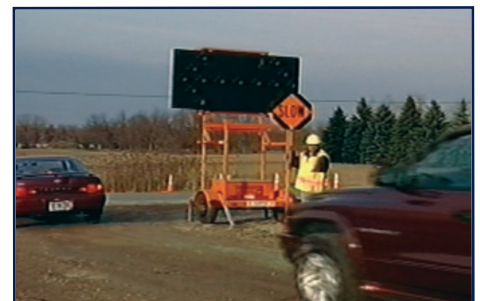
Flagging for road intersecting a TTC zone (Source: Michigan DOT).
