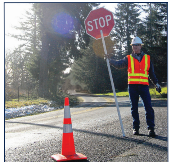
Flagger stopping traffic for temporary road closure ahead (Source: Washington State DOT).
