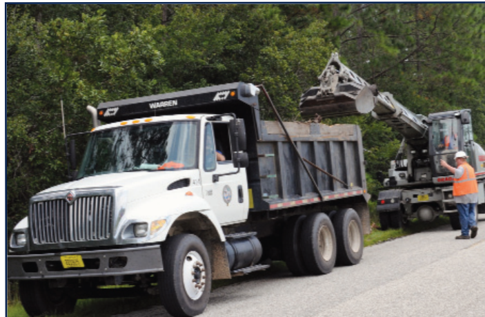
Example mobile work zone operation requiring flaggers (Source: G. Armstrong).
