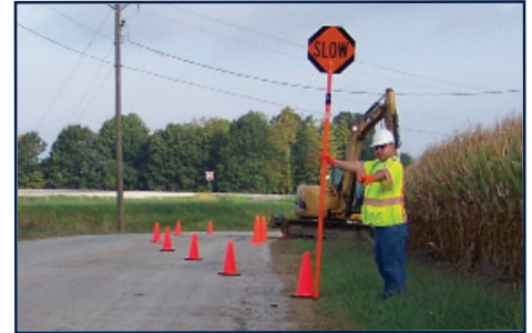
Example flagging operation on low-volume road (Source: N. Carboneau).
